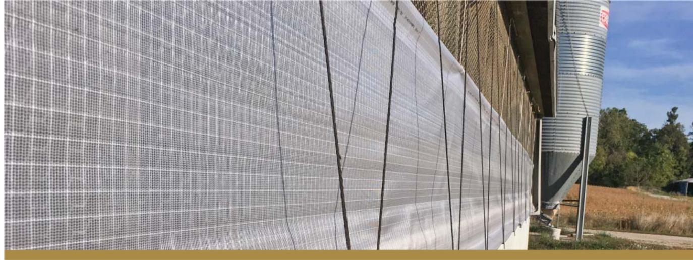
**DON'T:** Install the curtain when temperature is below 40° F (4° C).
